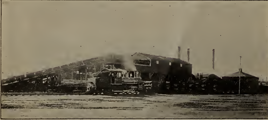
COLLIERIES AT WESTVILLE, NOVA SCOTIA.
